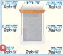
Install the bottom flashing over the wrap.
